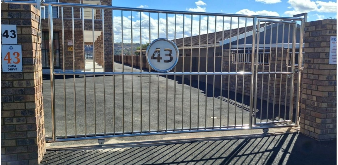
Custom stainless-steel gate with address feature
