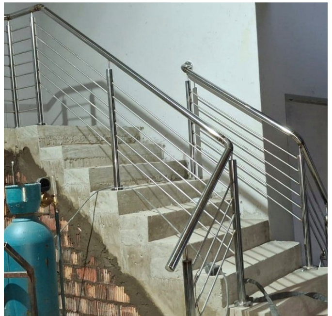
Multi-level stainless-steel handrail installation
