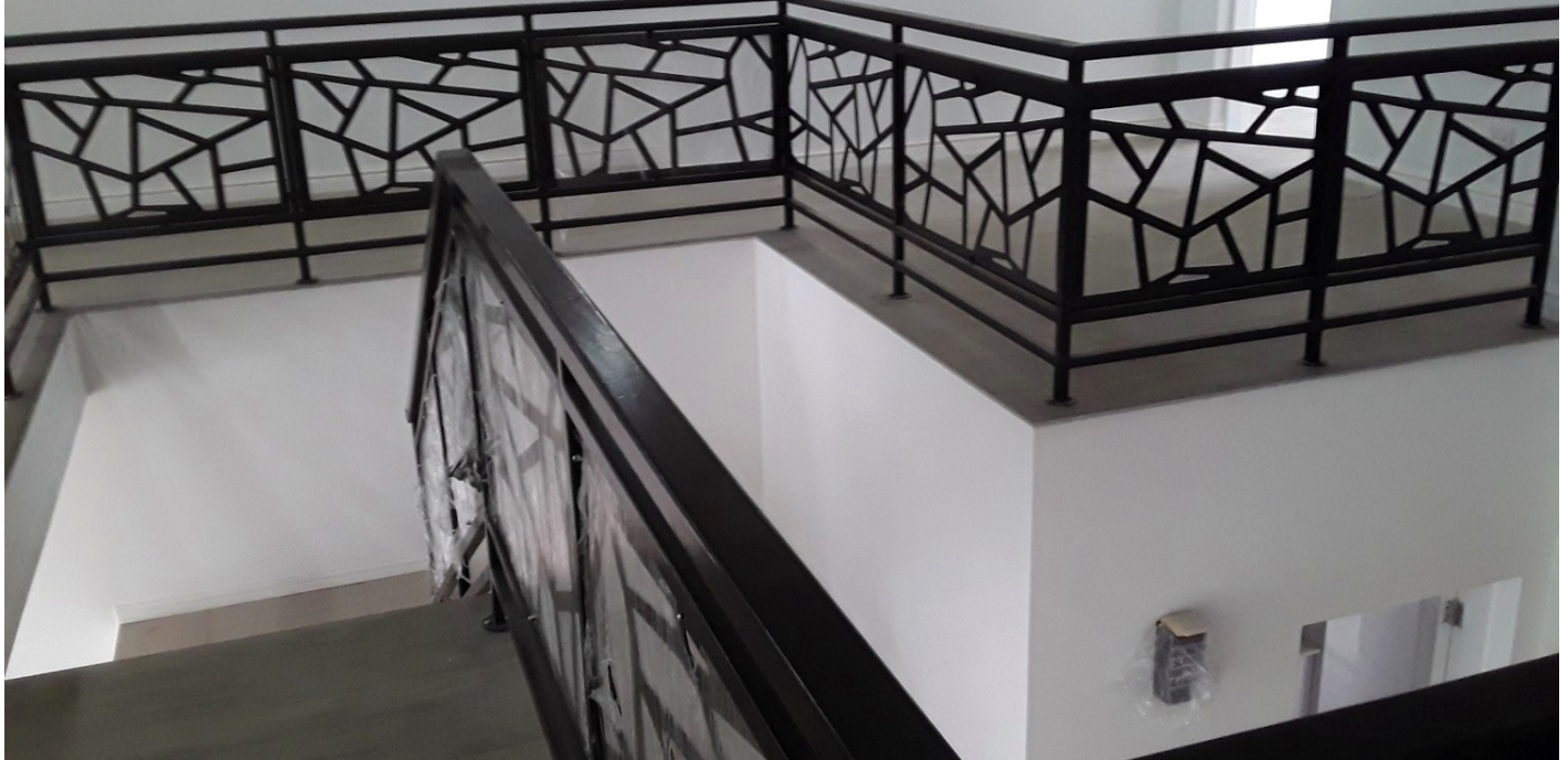
Coordinated railing around the stairwell
