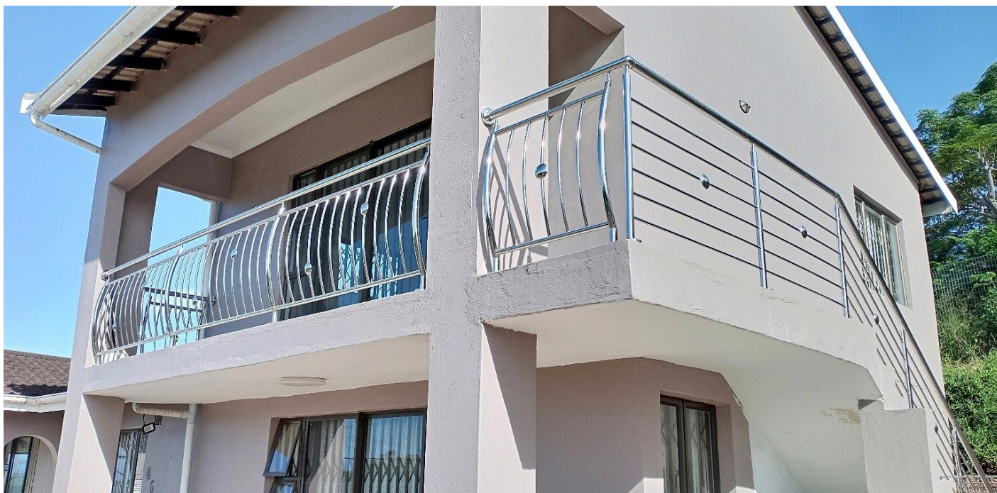
Curved and horizontal stainless-steel balcony balustrades
