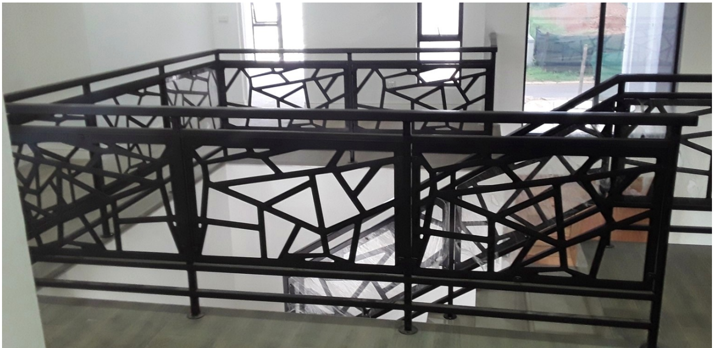
Completed geometric landing balustrade
