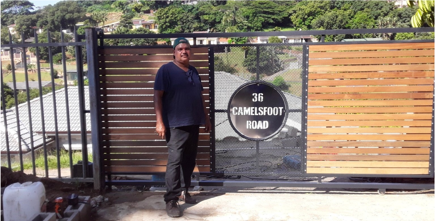
Custom sliding gate with timber and mesh infill
