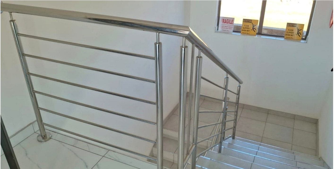
Interior stainless-steel stair and landing rails
