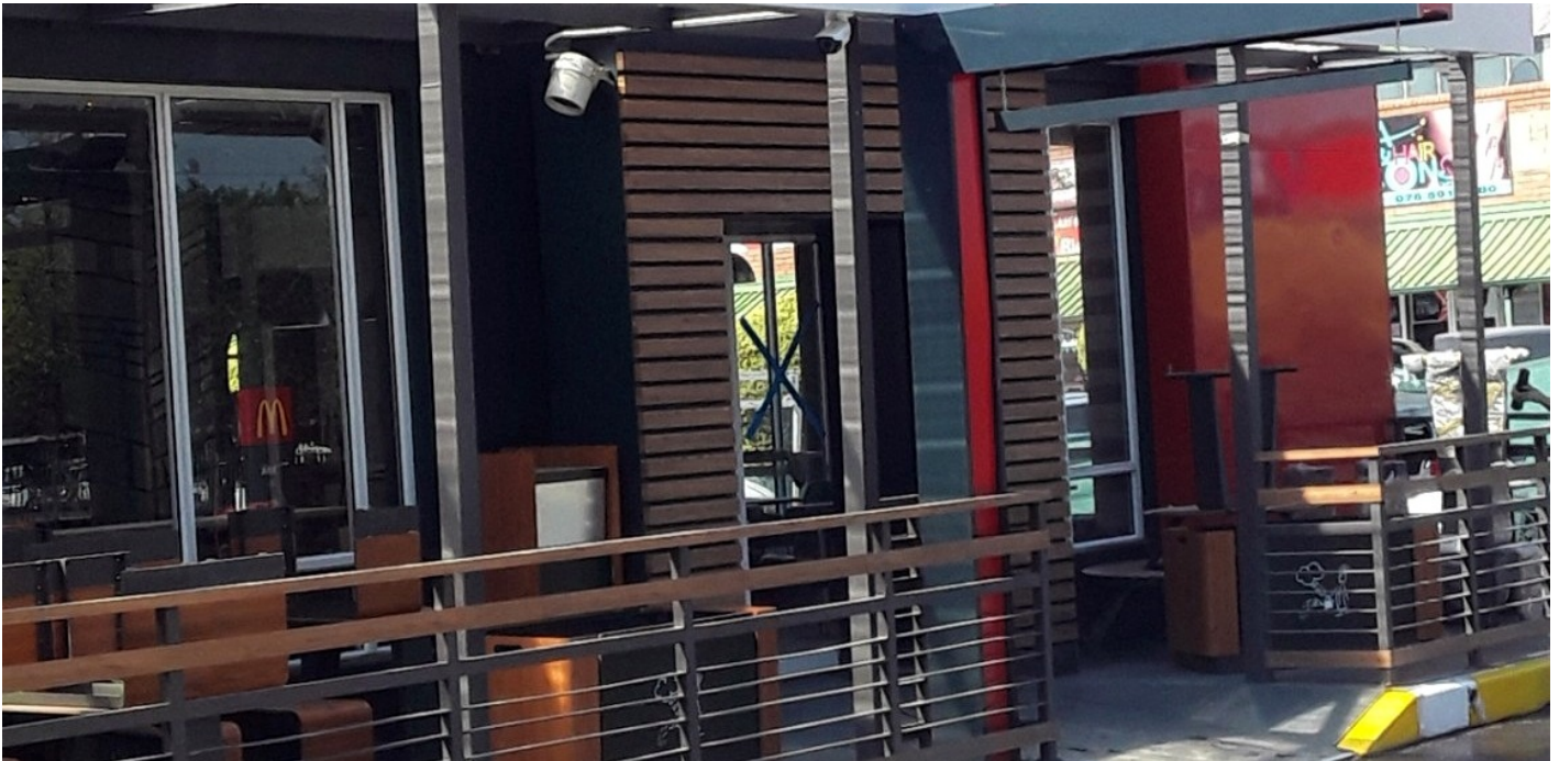
Completed commercial perimeter railing
