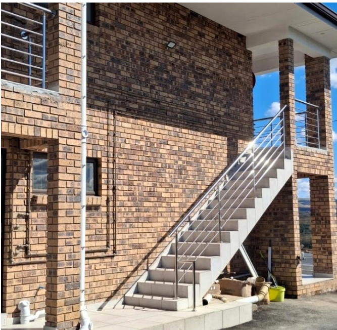
Exterior staircase balustrade
