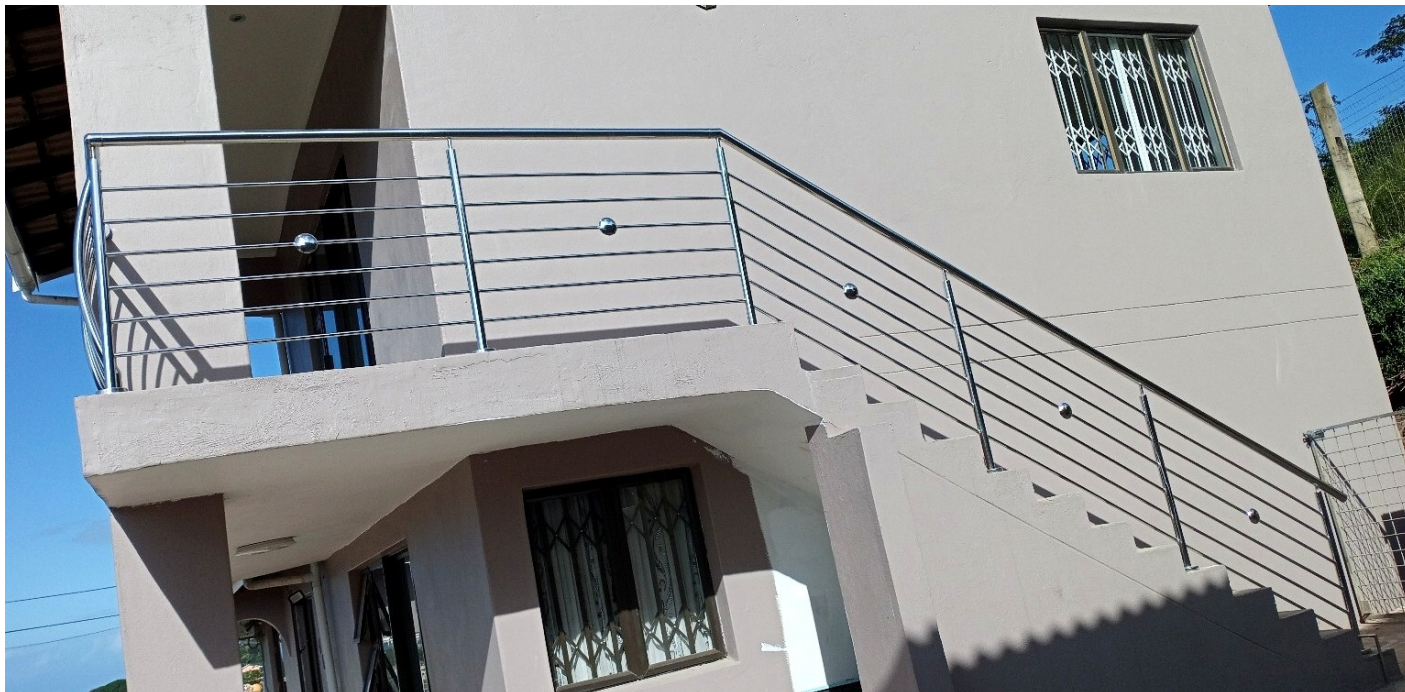
Stair and landing balustrade installation
