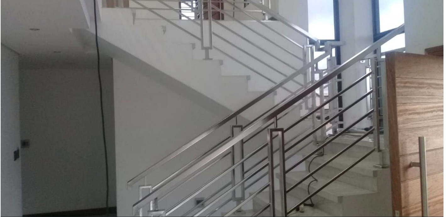
Multi-level interior staircase balustrade
