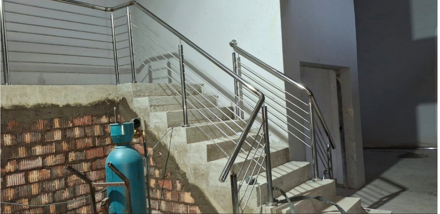
Fabricated rails fitted to a concrete staircase
