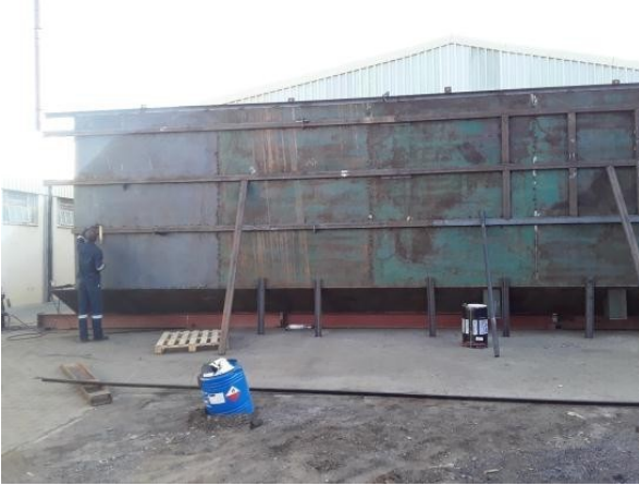
Fabricated industrial steel structure
