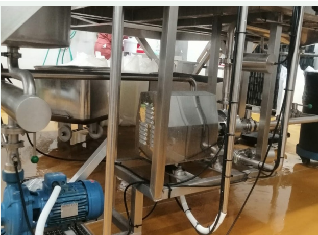
Pump, pipework and equipment installation
