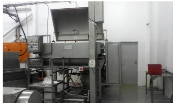
Food-production equipment installation
