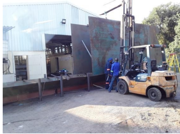
Structural installation in progress
