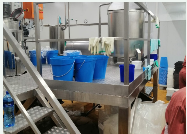
Access platform and stainless-steel vessels
