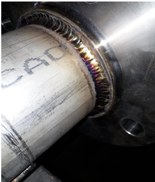
Stainless steel pipe welding
